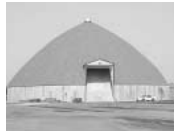
Finished dome shingled & full of salt.
