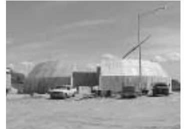
Setting the roof panels.
