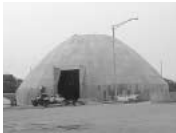
All roof panels set.
