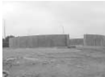
Finished concrete walls.
