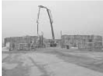
Pumping the concrete walls.
